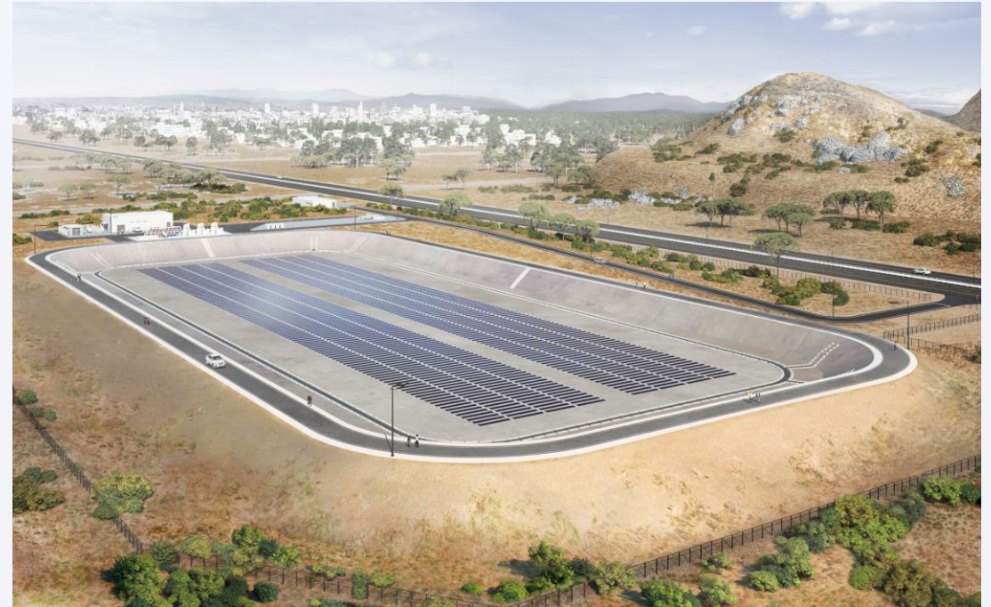
Water reservoir with Dynactive covering system (source: Benecke-Kaliko/Continental AG).
